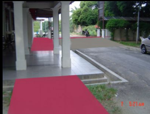
Slab Over Drain
