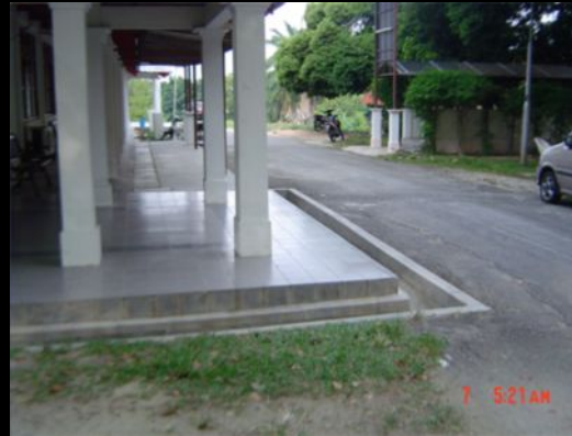
Slab Over Drain
