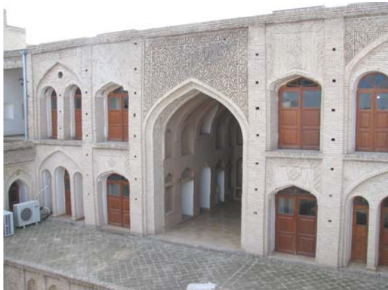
Figure 3. Iwan in a Traditional House Located in the City of Dezful, Southwestern Iran Source: Author
